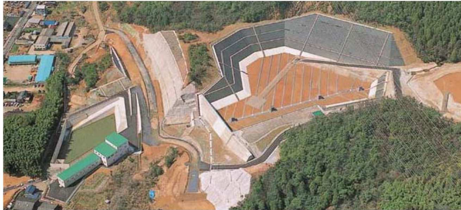
Final landfill/Facility for exudated water treatment
